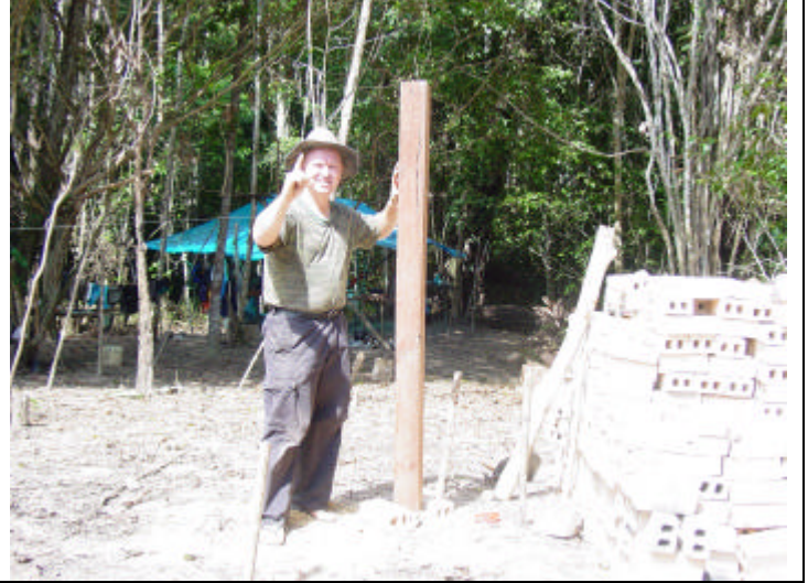
First Post of our house
