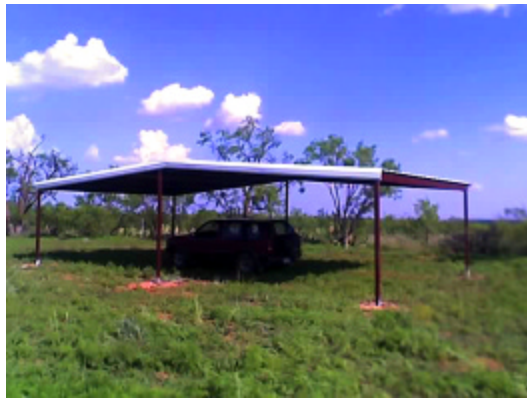
20X40 Roof (1 st structure of the Goff Ministries Camp)
