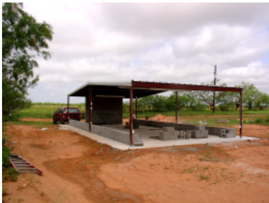
Main Abilene Camp structure Completed
